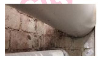
The debris/residue to walls behind redundant pipes in the switch room Z/002 does contain asbestos.
