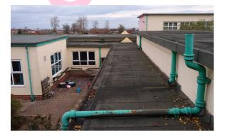
The flat roof (External Roof 8) does not contain asbestos.
