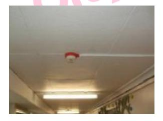
The ceiling board (Corridor 2/022) does not contain asbestos.
