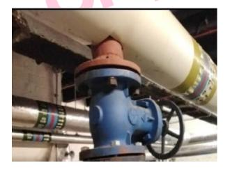
The pipework gaskets valve over boiler in the Boiler Room Z/001 does not contain asbestos.
