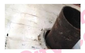
The debris/residue to wall redundant pipe area in the Boiler Room Z/001 does contain asbestos.
