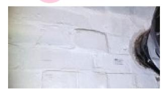
The debris/residue to wall adjacent to redundant pipe area in the Boiler Room Z/001 does contain asbestos.
