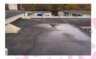
The flat roof (External Roof 4) does not contain asbestos.
