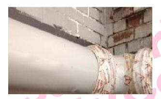
The pipework gaskets in the switch room Z/002 are presumed to contain asbestos.
