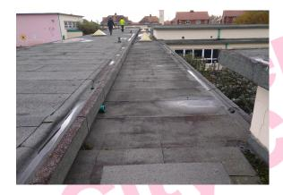
The flat roof (External Roof 15) does not contain asbestos.
