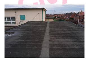
The flat roof (External Roof 3) does not contain asbestos.
