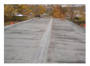
The flat roof (External Roof 10) does not contain asbestos.
