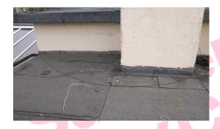
The sealant to flashing (External Roof 2) does not contain asbestos.
