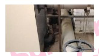
The debris/residue to floor behind boilers in the Boiler Room Z/001 does contain asbestos.
