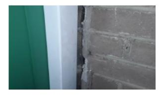
The damp proofing to doorframe in Kiln Room does not contain asbestos.
