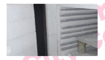
The vessel internal lining to kiln in Kiln Room does not contain asbestos.
