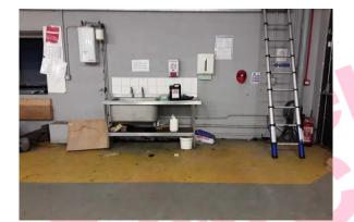
The sink pad to drainer (Area 1/Garage) contains asbestos.
