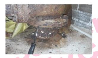
The metal flanges (bottom gasket) in Gas Meter cupboard do not contain asbestos.
