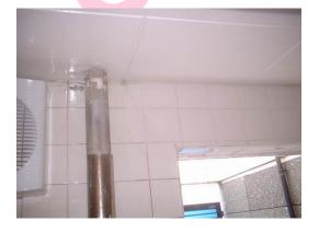
The flue to the kitchen (Room 0/67) contains asbestos.
