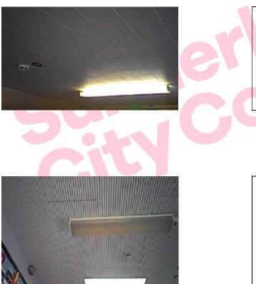
The suspended ceiling slats in Reception conservatory area does not contain asbestos.
