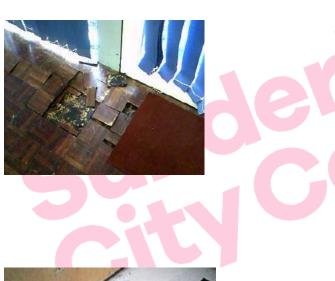
The parquet flooring and bitumen below in Key Stage 1 Hall does not contain asbestos.
