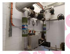
The pipework flange gasket where accessible (Rm 0/28 Reception Classroom) does not contain asbestos.
