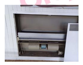
The panels behind heaters (Rm 0/29 Assembly Hall) contains asbestos.
