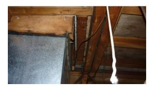
The central extraction duct lining in 0/32 Kitchen void above is presumed to contain asbestos.
