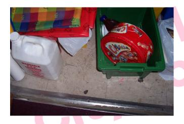
The white floor tiles and adhesive in area 4 (store cupboard) contain asbestos.
