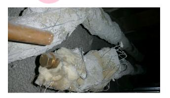
The firebreak & associated debris in 025/boys wc -void above does not contain asbestos.
