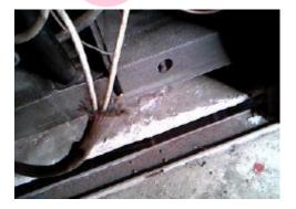
The rope to boiler 1 in Room 1 Boiler House does not contain asbestos.
