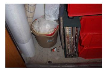
The white floor tiles and adhesive in area 5 (store cupboard) contain asbestos.
