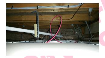
The firebreak & associated debris in 021/boys wc-void above does not contain asbestos.
