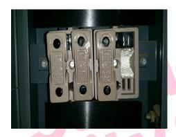
The flashguards within the distribution panel to the cupboard area (To become disabled WC) contained asbestos.
