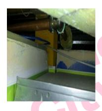
The insulating board cladding to the metal columns Classroom 6 (Room 13) contains asbestos.
