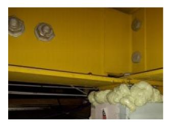
The lining to columns in the void above the Ladies toilets (Area 1) is presumed to contain asbestos.
