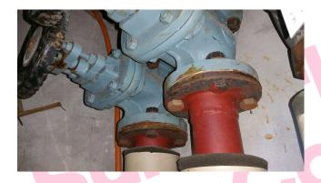
The Gasket to pipework flange (Rm 0/17) contains asbestos.
