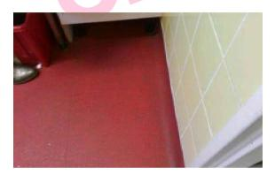
The skirting to base of wall in the store (Room 95) is presumed to contain asbestos.
