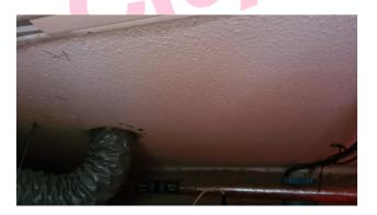
The textured coating to ceiling above suspended ceiling (G/013/Office) does not contain asbestos.
