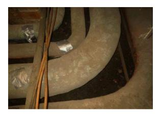
The large bore insulation – green pipework in the duct adjacent head teacher's office contains asbestos.
