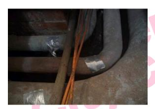
The small bore insulation – red pipework in the duct adjacent head teacher's office contains asbestos.
