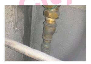
The debris on the pipework to the void to the upright heater in Year 1 room 6 does not contain asbestos.
