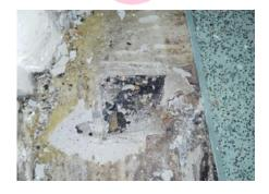
The composite floor (Area 5/Kitchen) does not contain asbestos.
