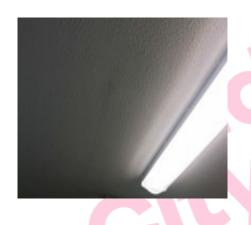
The textured coating to the ceiling in the kitchen (Room 002) contains asbestos.
