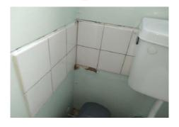
The adhesive behind ceramic tiles (Area 8/Staff WC) does not contain asbestos.
