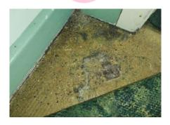
The composite floor (Area 2/Back Office) does not contain asbestos.
