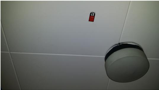
The ceiling in Rm 008/reception contains asbestos.
