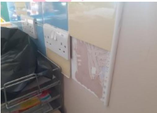
The walls rear of ceramic tiles adhesive in Kitchen within reception area do not contain asbestos.
