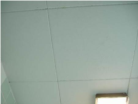
The ceiling tiles to the male toilets (Rm 0/09) are presumed to contain asbestos.
