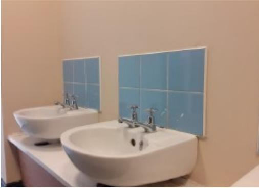
The walls rear of ceramic tiles adhesive in Reception WC Area do not contain asbestos.
