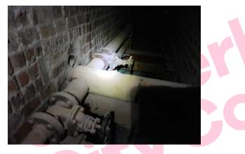
The pipes (Gaskets) (Area 4/Loft Space 4) are presumed to contain asbestos.
